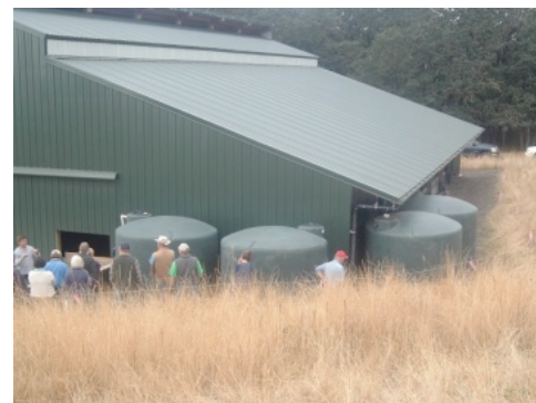
These four 2,500 gallon water harvesting tanks capture rainwater from the barn's roof and help save over 162,000 gallons of water a year that would otherwise be pumped from the groundwater aquifer below. Photo courtesy of Yamhill Soil & Water Conservation District.
