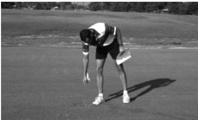
Flag each sprinkler head. Use a different color of flag for each zone.
